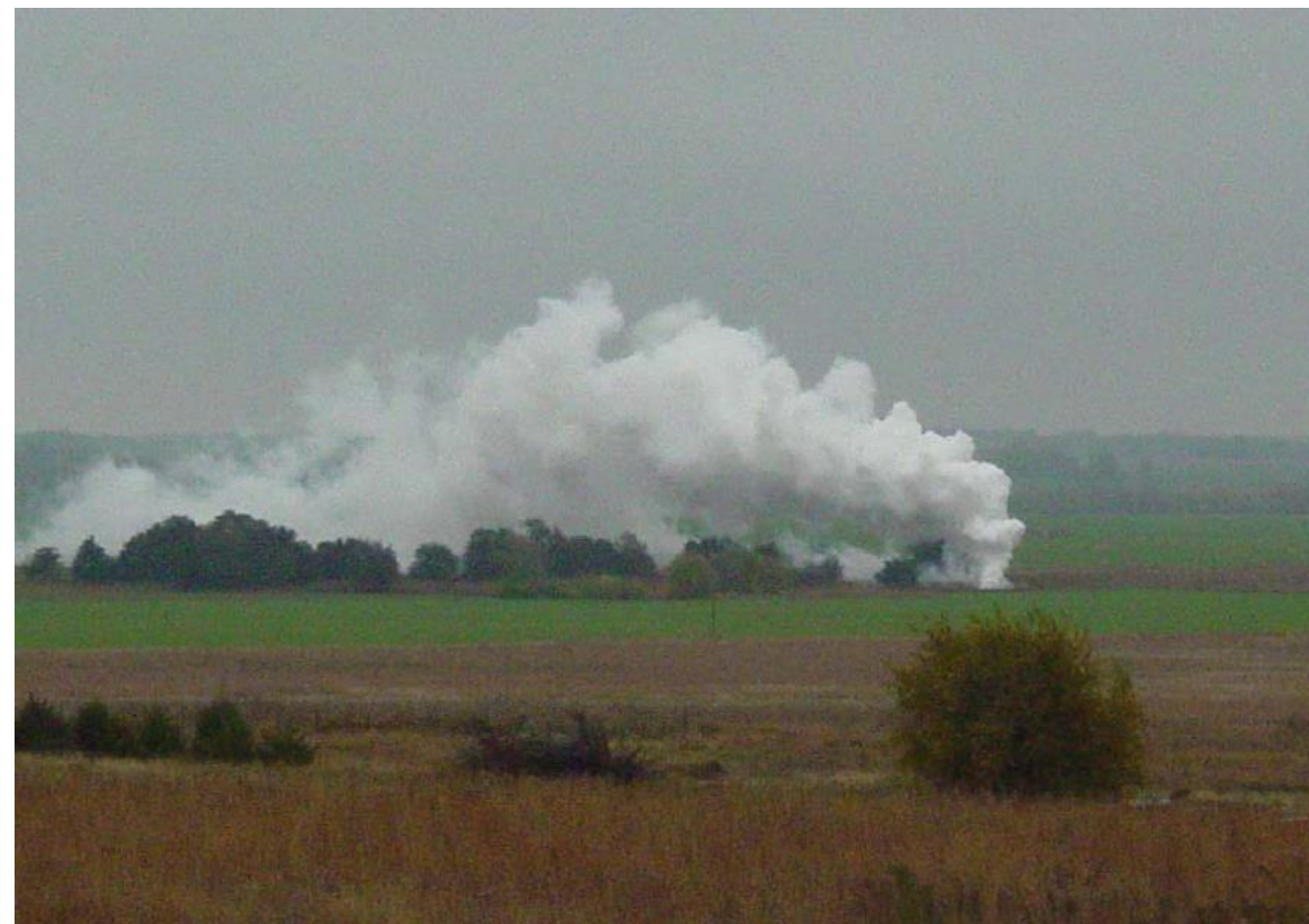
Ammonia pipeline release, Kingman, Kansas (2004)
