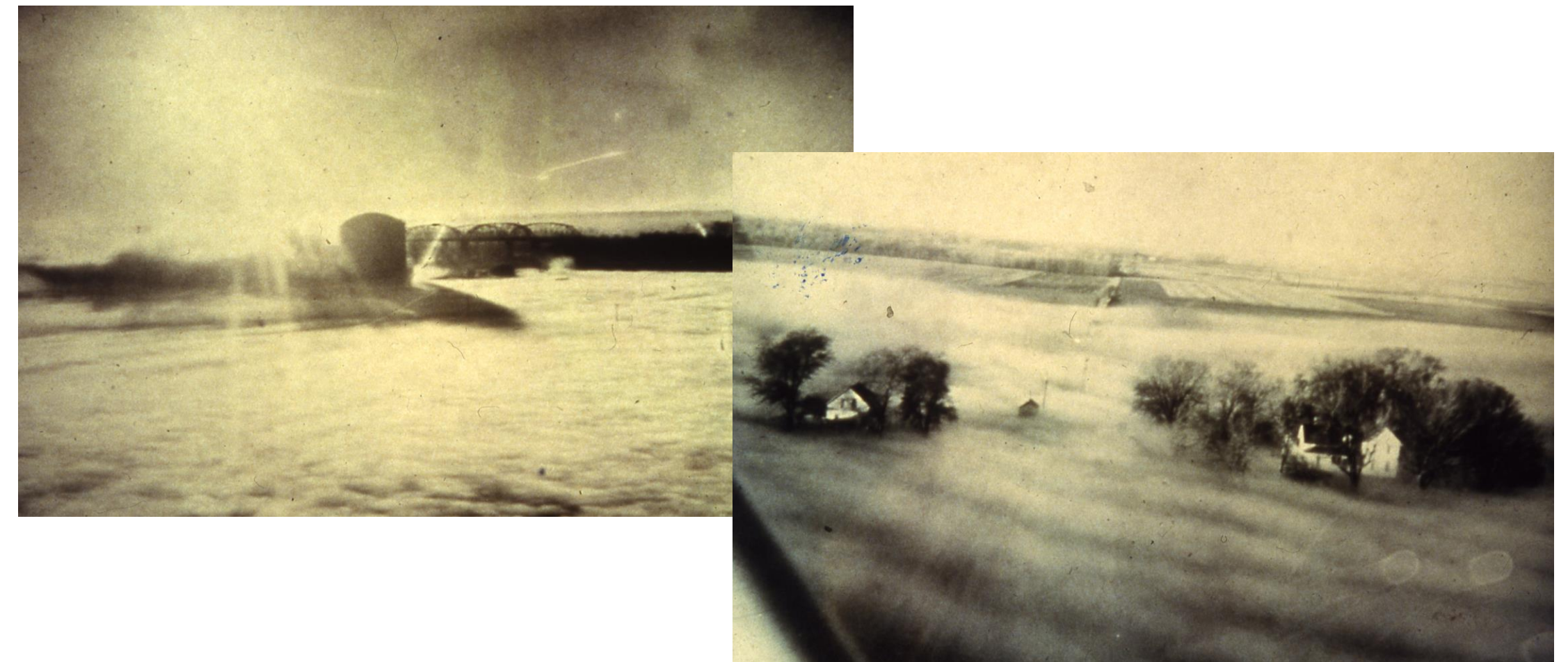
Ammonia storage tank overfilling, Blair, Nebraska (1970)
